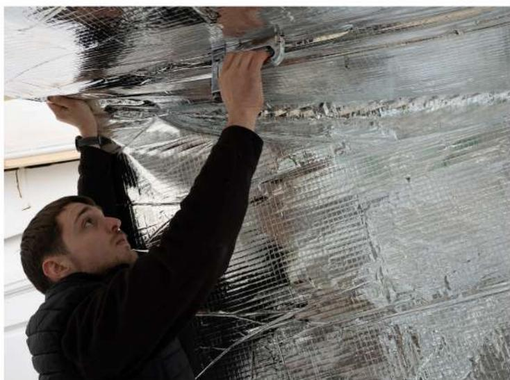
The next step is to roll out the insulation to the desired length and cut using a sharp blade or multifoil scissors. Lift insulation up to the battens and staple onto the battens as a taut continuous layer across the roof area. This will have created the required air cavity between the roof and insulation.
