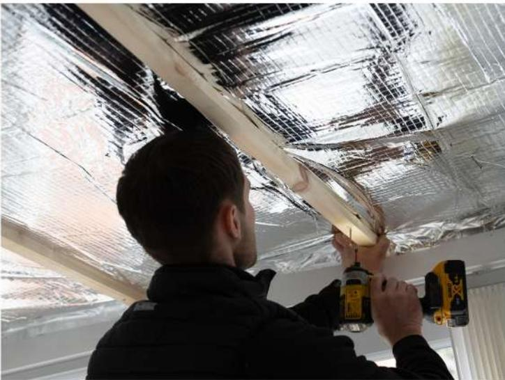
The next step is to install 25mm counter battens over the insulation. We recommend using the FastFix Multifoil Screws at 300mm intervals. This will compress the insulation down to just 5mm, taking up minimal roof height. The battens can be installed either vertically or horizontally.
