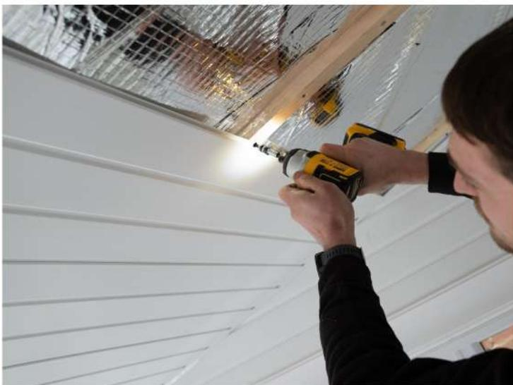
The next step is to measure and cut the Conservaclad boards to size. These can be installed by sliding the boards into the ConservaClad end caps around the perimeter and screw into the battens using 10mm+ Dry Wall Screws. We recommend to start at the bottom of the conservatory and work your way up. The ConservaClad Boards are connected together using a tongue and groove system.
